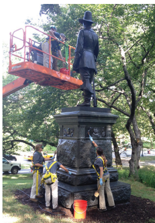
Conservation Technicians at work on The Pilgrim.
